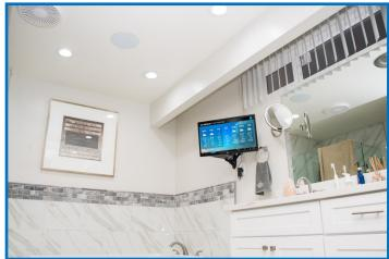
For ultimate convenience a variety of wall switches, keypads, and dimmers were installed to control 20 separate lighting loads. In addition to lighting, wall keypads also control fireplaces, thermostats, speakers, TVs, and alarm system. With one touch the customer can trigger a number of preset scenes such as:
