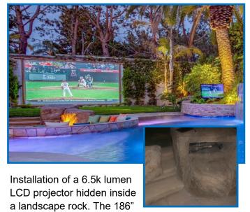
screen was painted on the wall with specialized contrast paint. Every square foot of the backyard has a clear view of the screen. The projector is on a video matrix and is controlled using the automation system.
