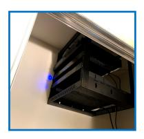
All wires were ran to the headend room. Installation of a rack containing the network, video recorder, power conditioner, and cooling system.
