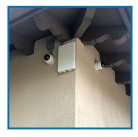
Two additional all weather access points were surface mounted to the exterior of the house for quality Wi-Fi coverage throughout the grounds.
