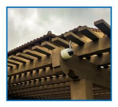
A vandal dome camera with cabling running through conduit to a patio cover.
