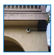
12 vandal dome cameras were installed on the exterior of the house to cover the grounds.
